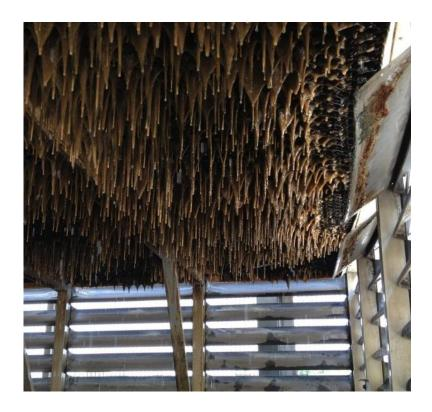
Because of biofilm build up on the surface a dramatic drop in efficiency occur. It has been shown that the efficiency typically can be reduced with up to 15%, above picture illustrate how a cooling tower can harbor biofilm. A reduction of efficiency is obviously.
